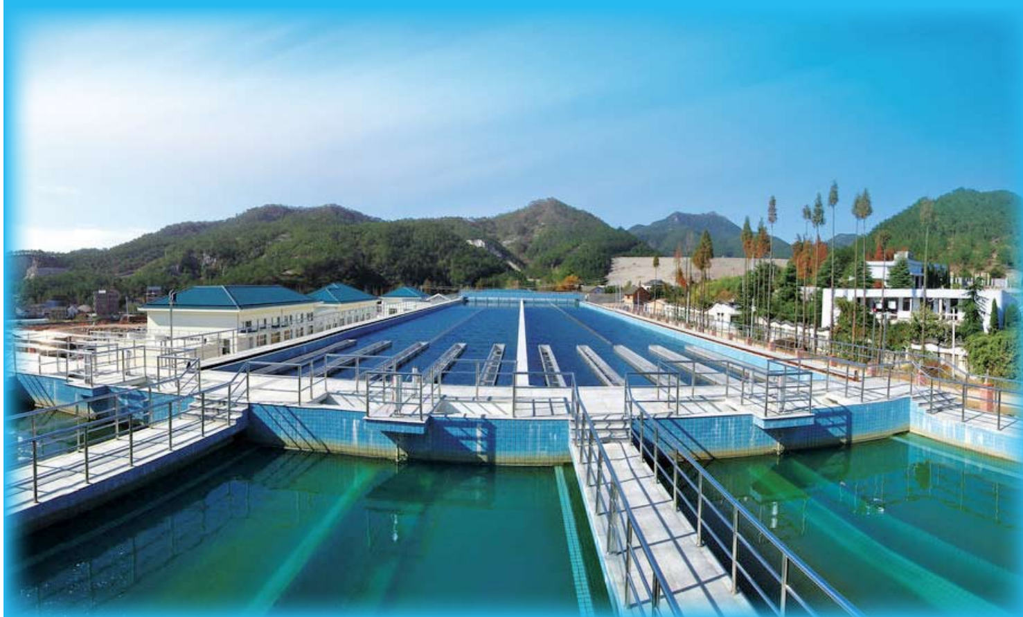
Weifang City Tap Water Supply 潍坊自来水供水
