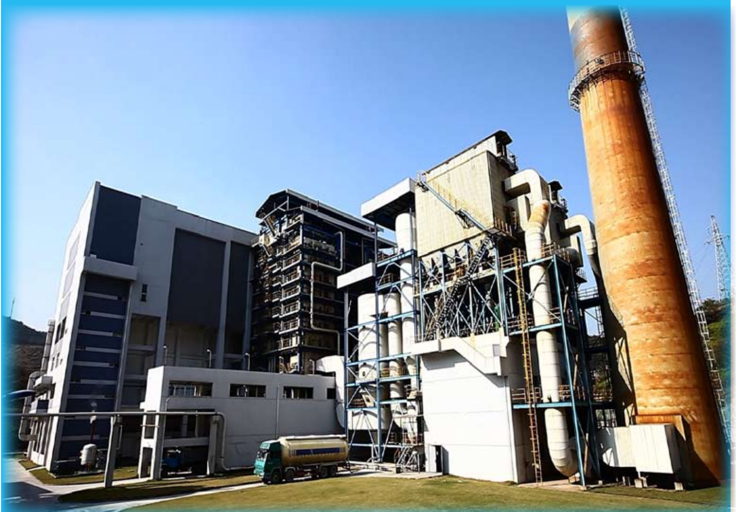
Wenling Waste Incineration Power Generation 温岭固废发电
