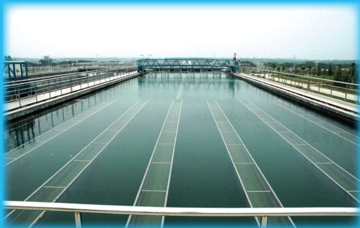
Weifang City Tap Water Supply 潍坊自来水供水
