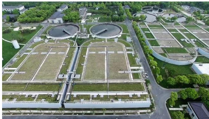
Figure 8. Qingpu Second Wastewater Treatment Plant Project (Expansion).
