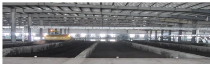
Figure 13. Bioleached and dewatered sludge at one of our Northeast China wastewater treatment plants.
