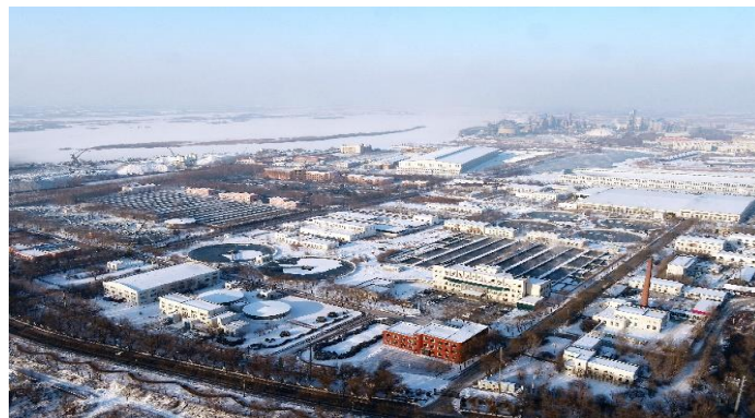
Figure 7. Harbin City Wenchang Taiping Wastewater Treatment Plant.
