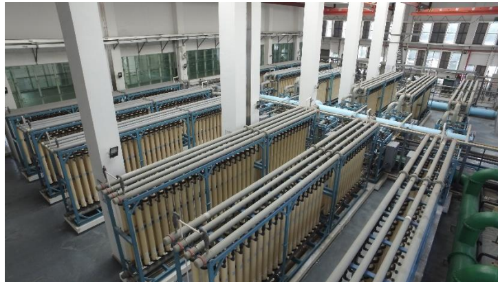
Figure 10. Advanced ultrafiltration membranes used for wastewater treatment at one of our South China reclaimed water plants.
