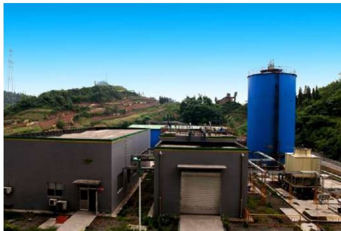
Figure 14. Wastewater treatment system at the Dazhou City Municipal Household Waste Incineration Power Generation Project 1st Phase.
