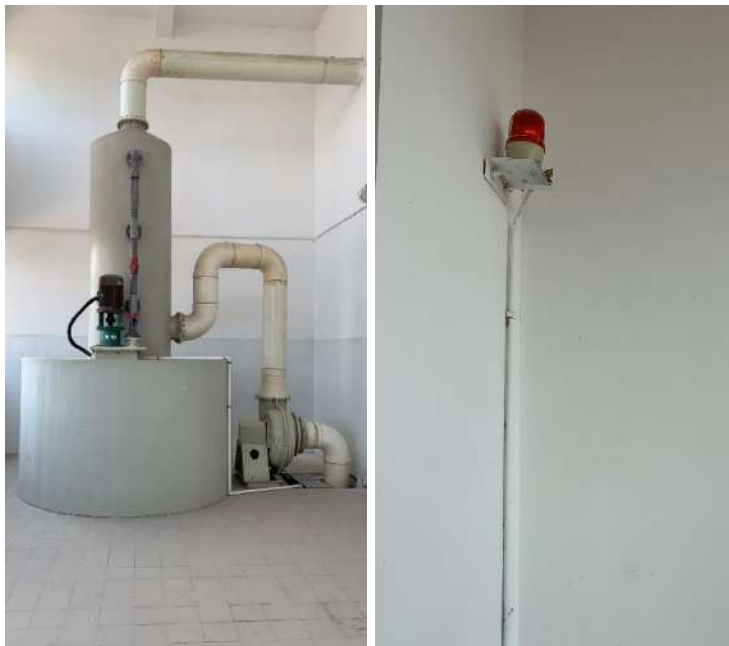
Figure 7. Chlorine gas absorption device (left picture) and alarm system (right picture) at a water treatment plant from our Central China business unit.
