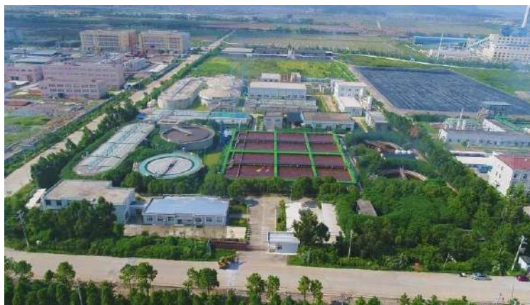
Figure 4. Linhai Park WWTP Project with high rates of foliage coverage purifying the site.
