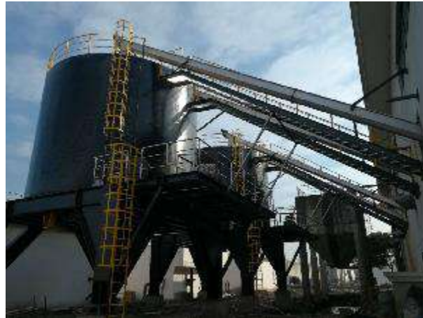
Figure 8. Sludge chamber of a project under the East China business unit.
