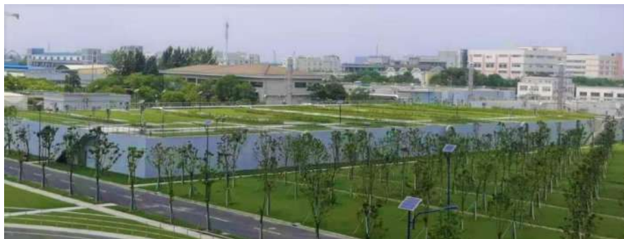
Figure 3. Qingpu Second WWTP Project 4th Phase (Expansion) grow plants on top of the cover to help purify the air and reduce the impact of odorous gas on the surrounding environment.
