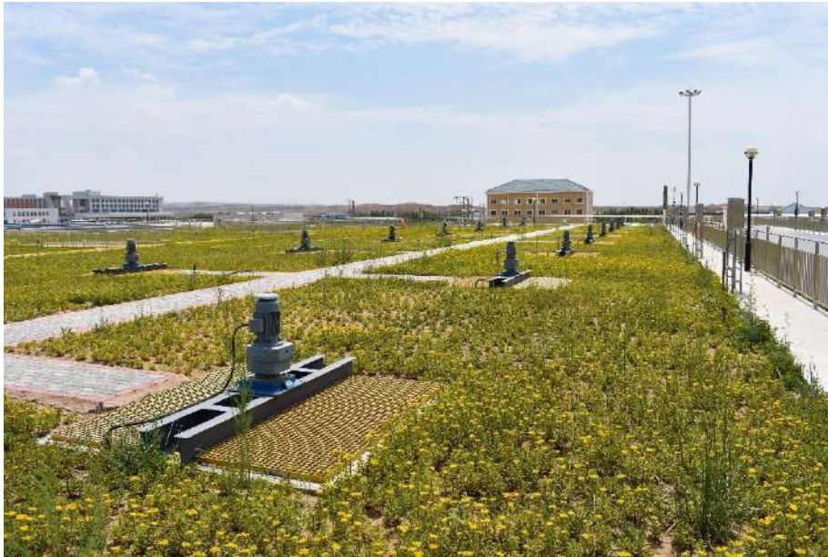
Figure 2. Yinchuan Binhe District WWTP Project 1st Phase covers the biological treatment units.
