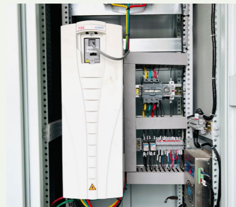
Submersible pumps in the lift pump room were equipped with frequency converters to meet energy saving requirements
