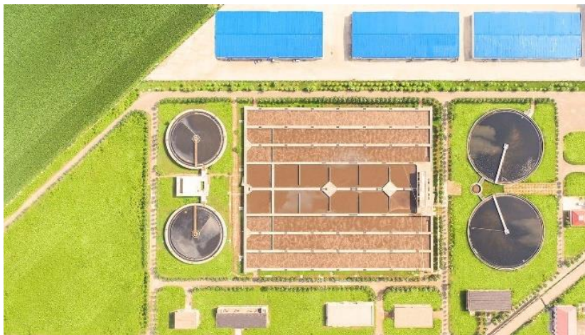
Figure 15: Harbin City Xinyi Wastewater Treatment Plant
