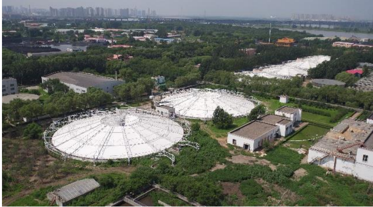
Figure 8: Sewage deodorisation facilities
