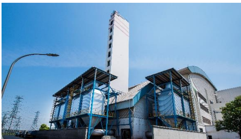
Figure 7: Activated carbon adsorption tower
