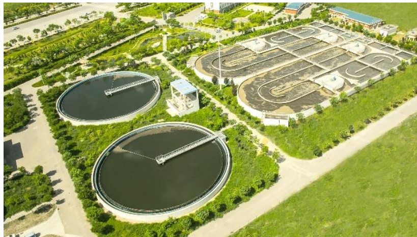
Figure 16: Yinchuan Wastewater Treatment Fifth Water Reclamation Plant
