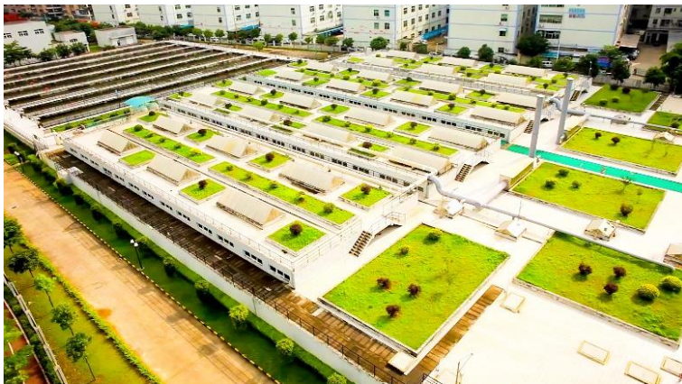
Figure 10: Deodorisation system at our Shenzhen Henggang Wastewater Treatment Plant
