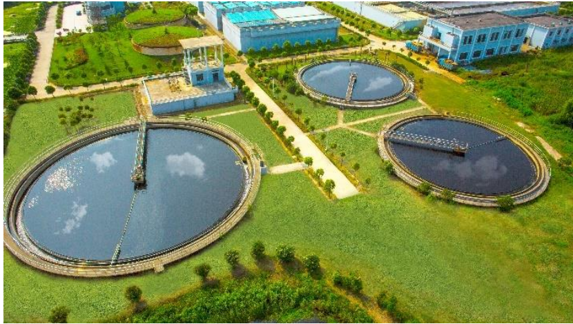
Figure 14: Ningbo Hangzhouwan New District Wastewater Treatment Plant
