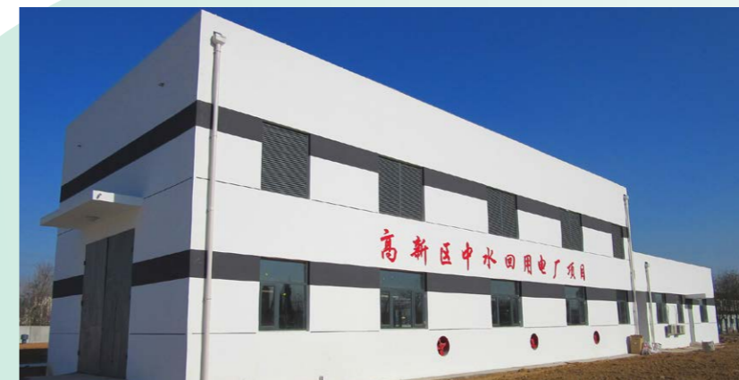
Reclaimed water pump room of North BU
