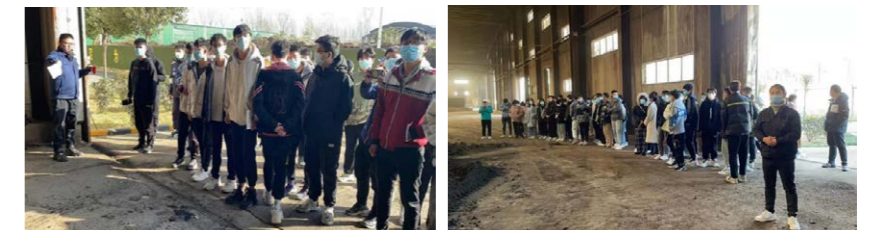
Teachers and students of Nanyang Institute of Technology visited Nanyang Zhonghui Sludge Treatment and Resource Utilisation Project
